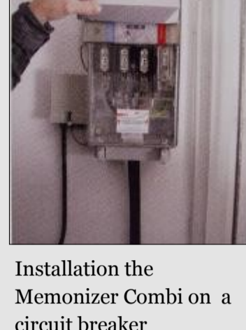
Installation the Memonizer Combi on a circuit breaker
