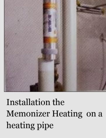
Installation the Memonizer Heating on a heating pipe
