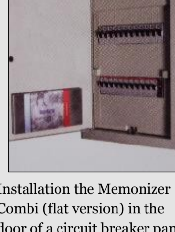
Installation the Memonizer Combi (flat version) in the door of a circuit breaker panel
