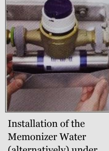
Installation of the Memonizer Water (alternatively) under the water meter
