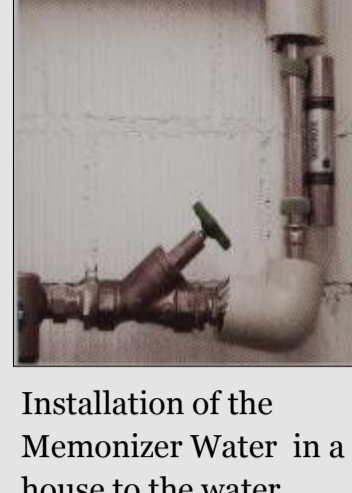
Installation of the Memonizer Water in a house to the water pipes in the cellar
